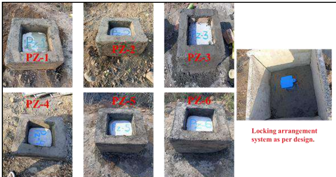
Figure 22: Preparation of concrete platform and locking arrangement for the piezometers (PZ-1 to PZ-6) installed around the ash dyke of NTPC Khargone
