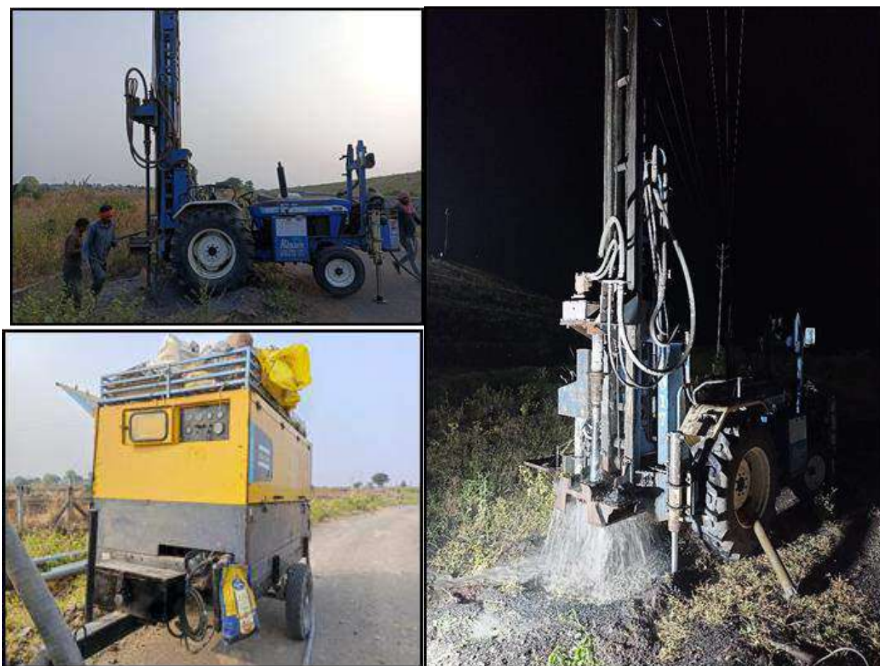
Figure 19: Drilling operation in progress for construction of the piezometers around new Ash Dyke, NTPC Khargone
