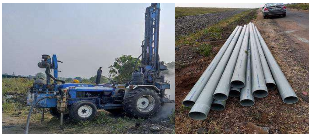
Figure 20: Cleaning of borehole using air compressor, supply and installation of 5-inch casing (PVC) pipe in progress for construction of the piezometers around ash dyke at NTPC Khargone.
