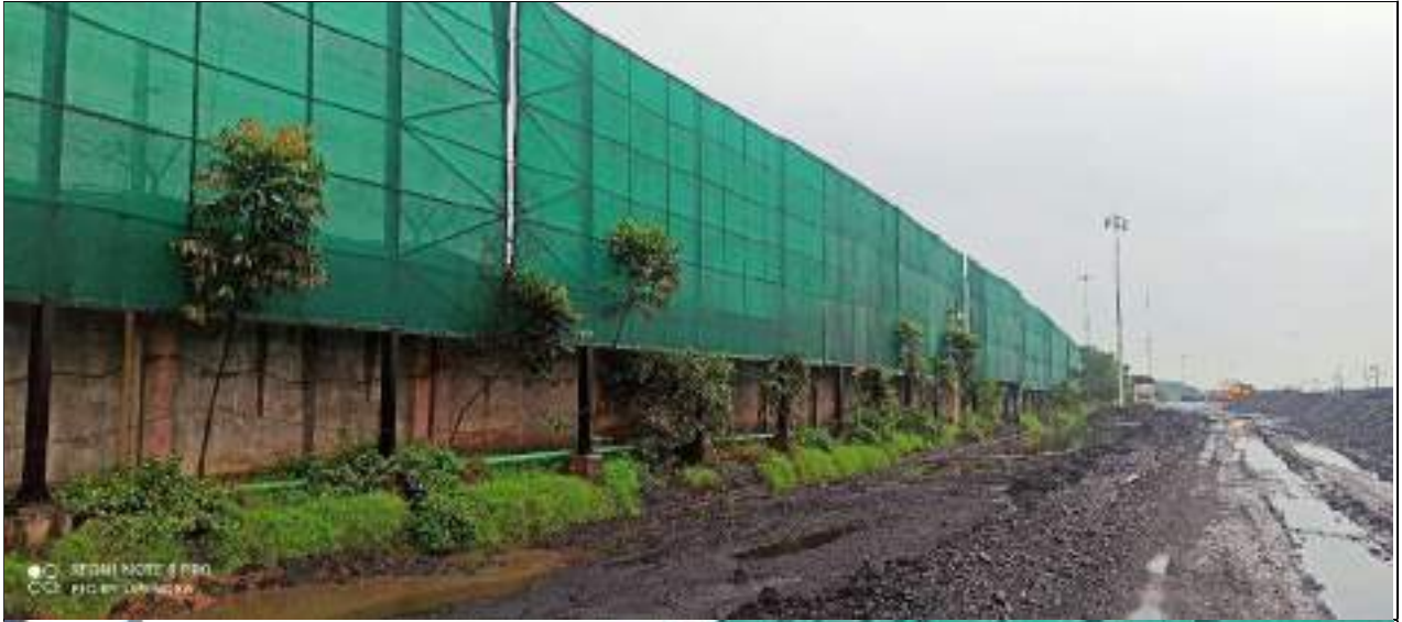
Photographs of Boundary wall with 20 ft. windscreen
