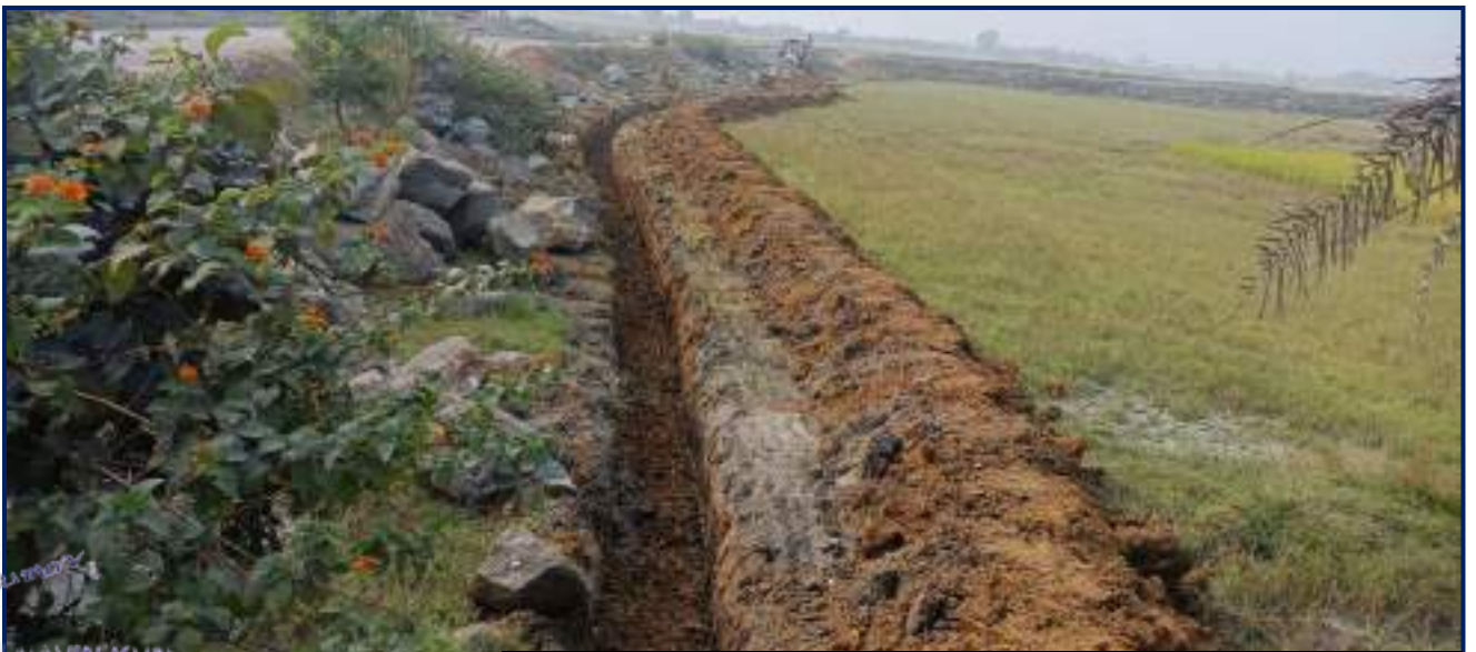
Garland Drain & Catch Drain along Top Soil & Embankment
