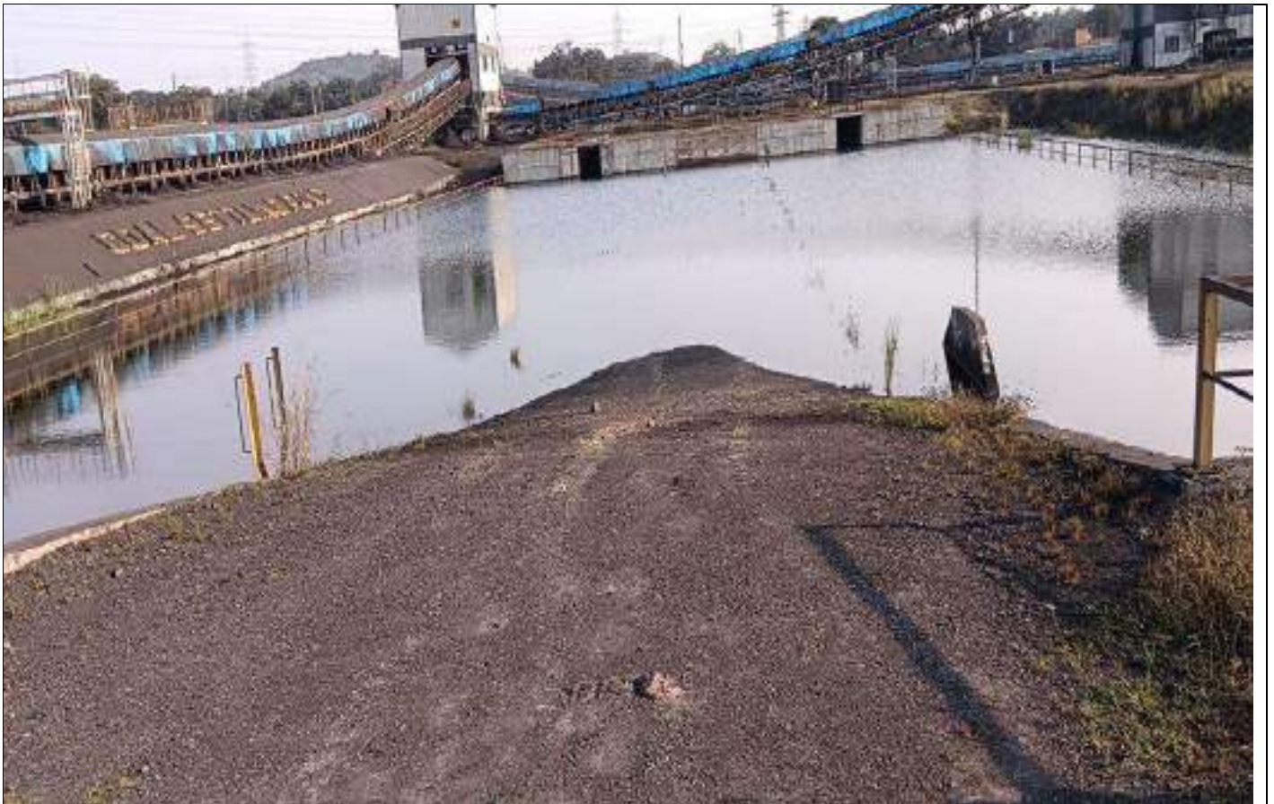
PHOTOGRAPH OF SETTLING TANK AT CHP AREA
