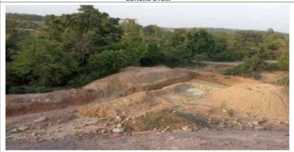
Garland Drain connected to settling pond
