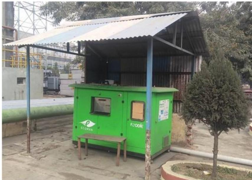
125 kg/day capacity Organic Waste composting ‘FOODIE’ machine has been installed for sustainable management of biodegradable waste generated from plant canteen.
