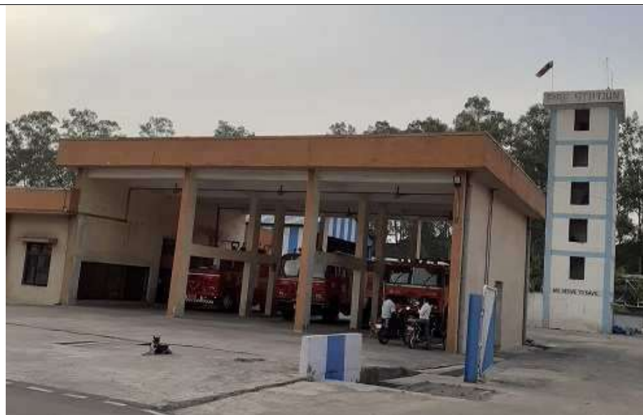
NTPC Vindhyachal Fully equipped CISF manned central fire control station
