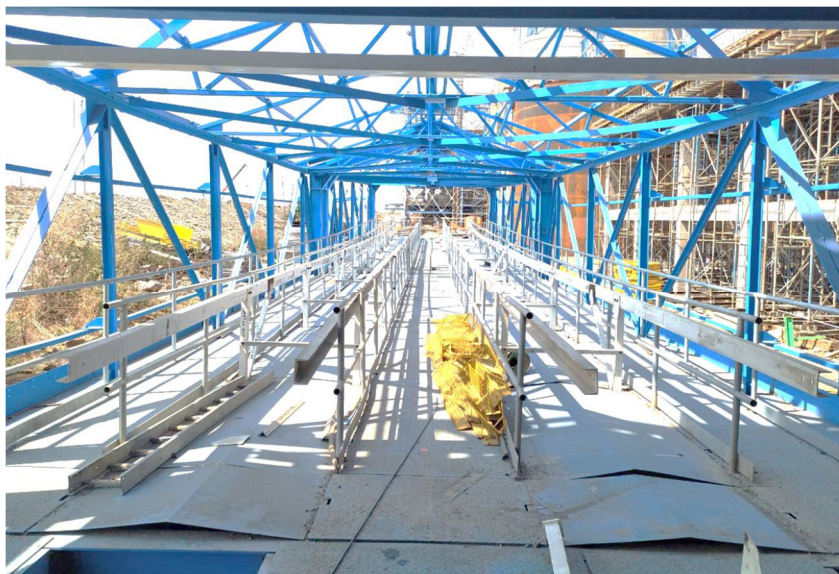
Limestone Handling System Conveyor gallery
