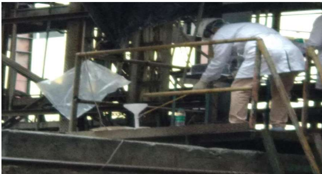
Figure 8: Injecting the fly ash in the slurry tank through funnel
