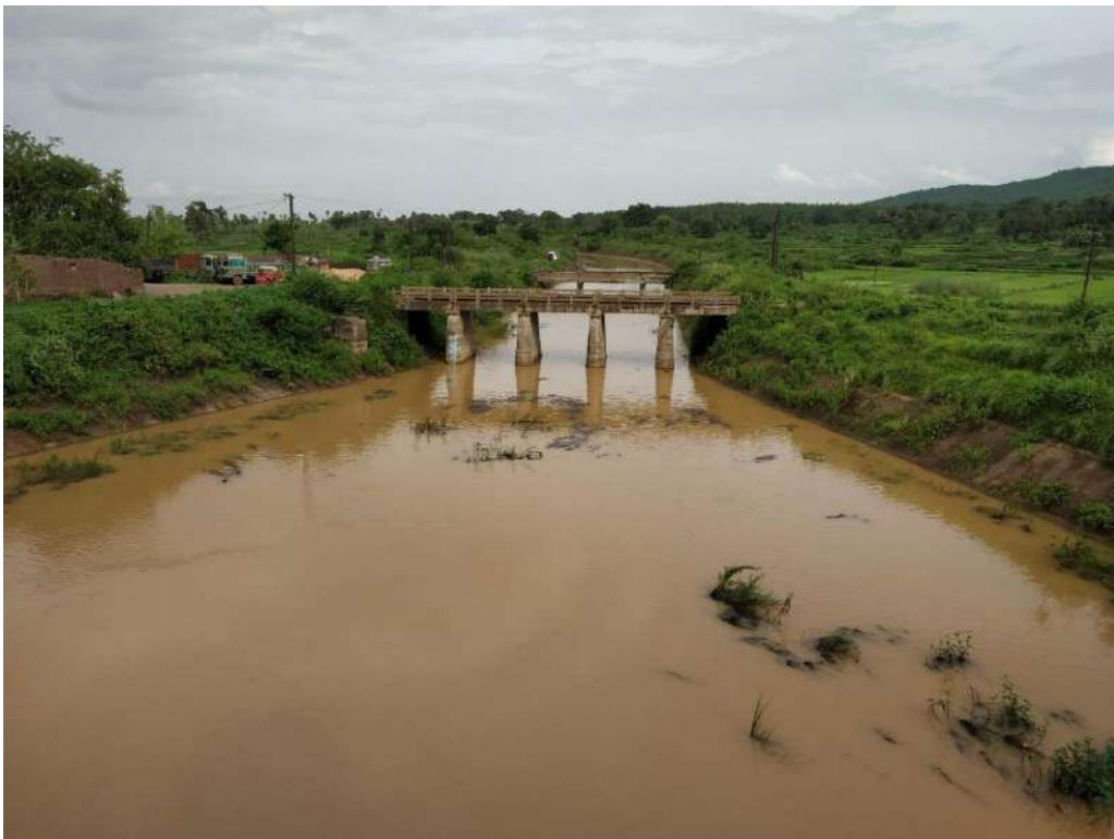
Fig. 3.7 Right Bank Canal from Samal Barrage (TTPS Stage III intake is proposed along this canal)
