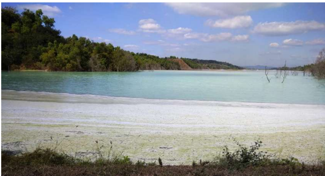
Figure 3: decantation zone from where water is recycled to the plant
