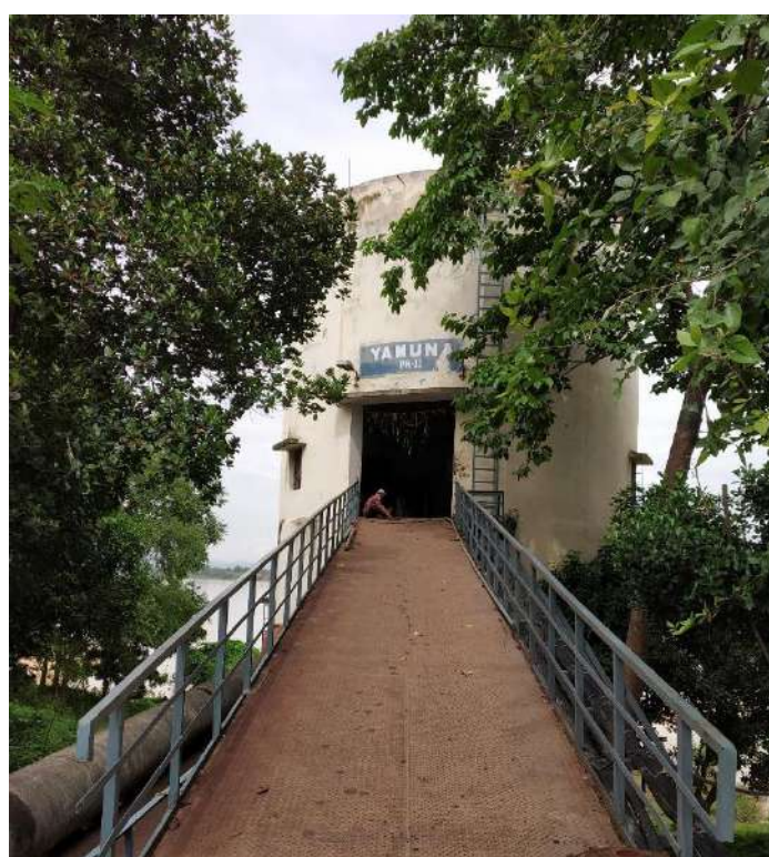
Fig. 3.5 Intake Pump House of MCL, Talcher
