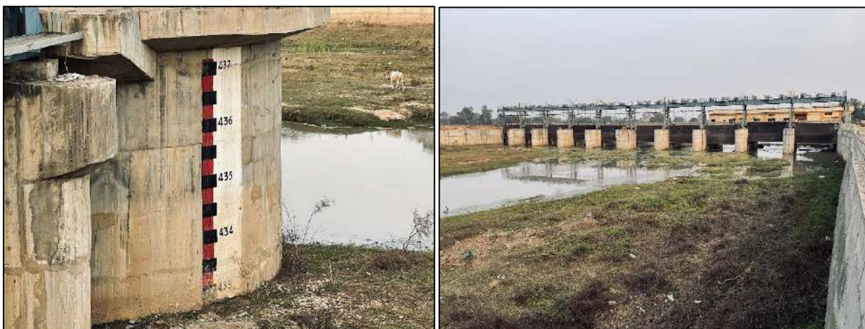
Fig. 4. Site photograph of water level gauge and check dam on January 25, 2021.
