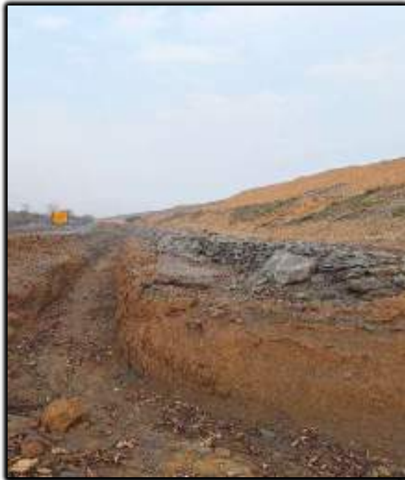
Picture: Construction of Garland Drain & toe wall along dump i/p
