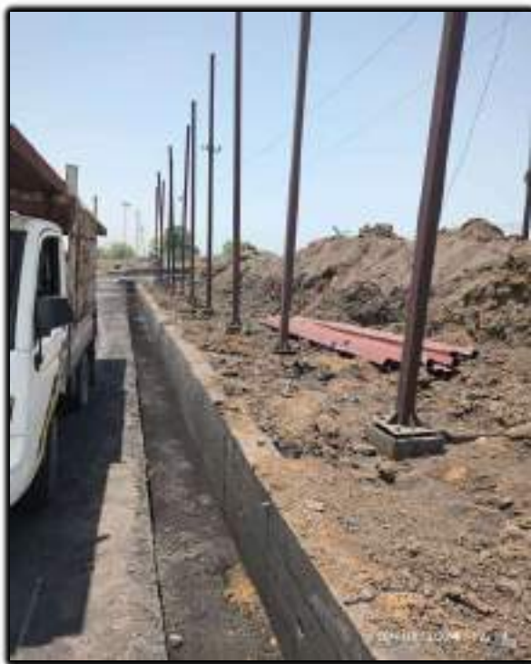
Picture: Construction of Garland Drain & toe wall along dump i/p
