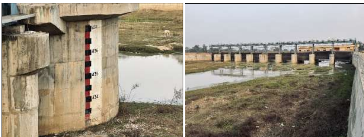
Figure 12. Site photograph of water level gauge and check dam on January 25, 2021, during the pre-monsoon period (1 st year).
