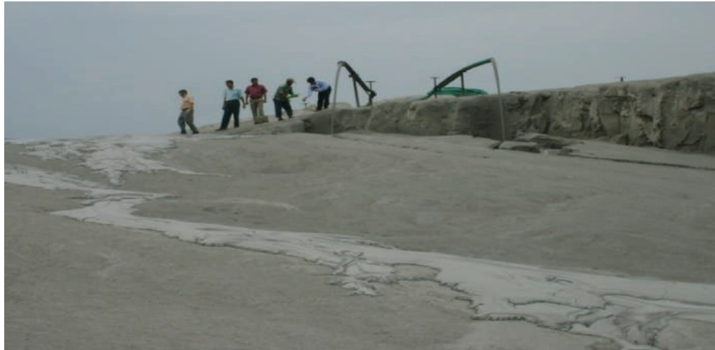
Plate-5.4: High Concentration Slurry Flowing on Slopes which dries out by the time it travels 30-40 m from the source
