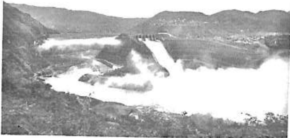
Photograph showing the passage of floods over the ski jump
