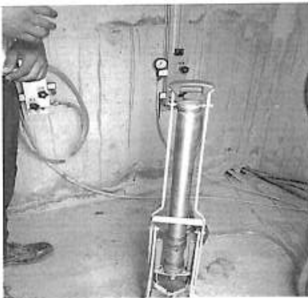
Cell Settlement System in the Dam Body on the Downstream Side
