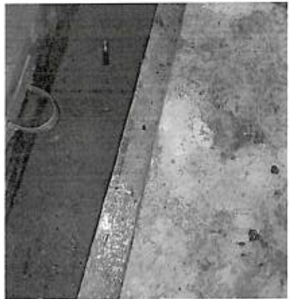
Automatic Water Level Measurement in Drain
