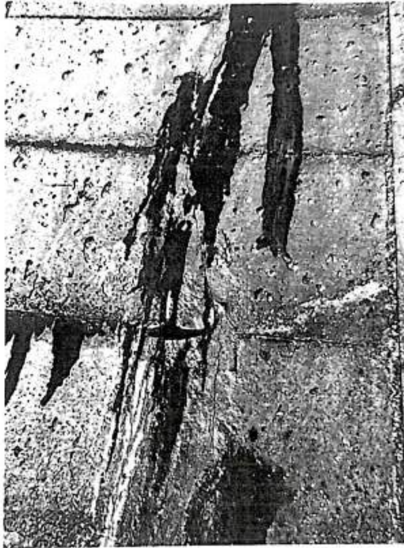
Photo 3 : PU grout filled in the cracks, covered with plaster
