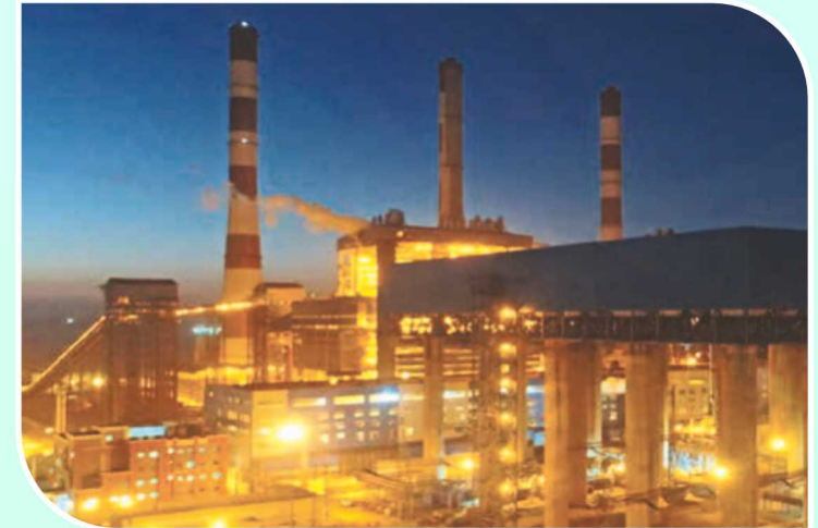
Air Cooled- Condenser at NTPC Patratu
