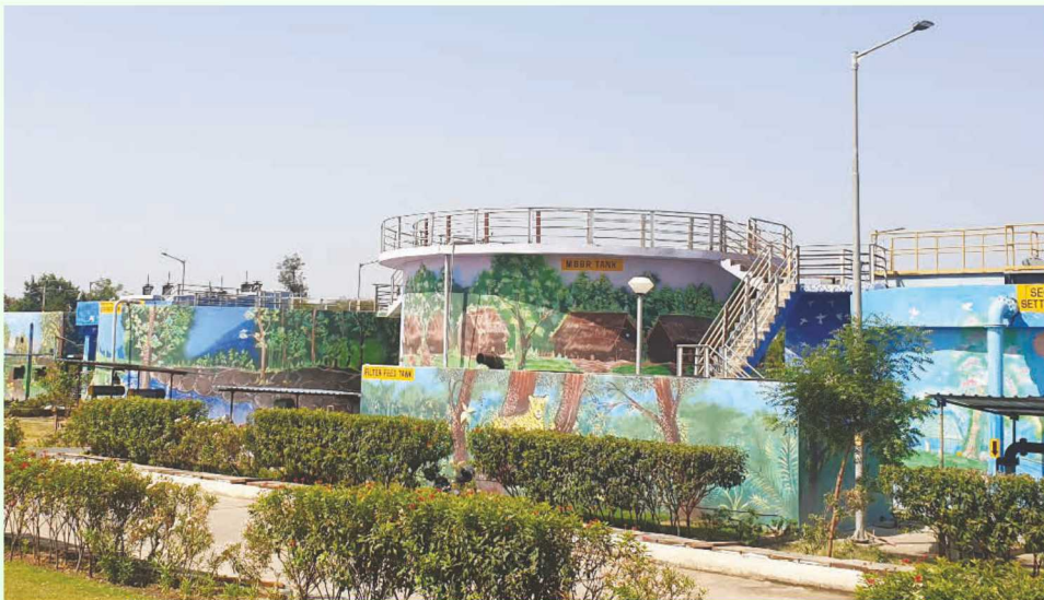
Sewage Treatment Plant
