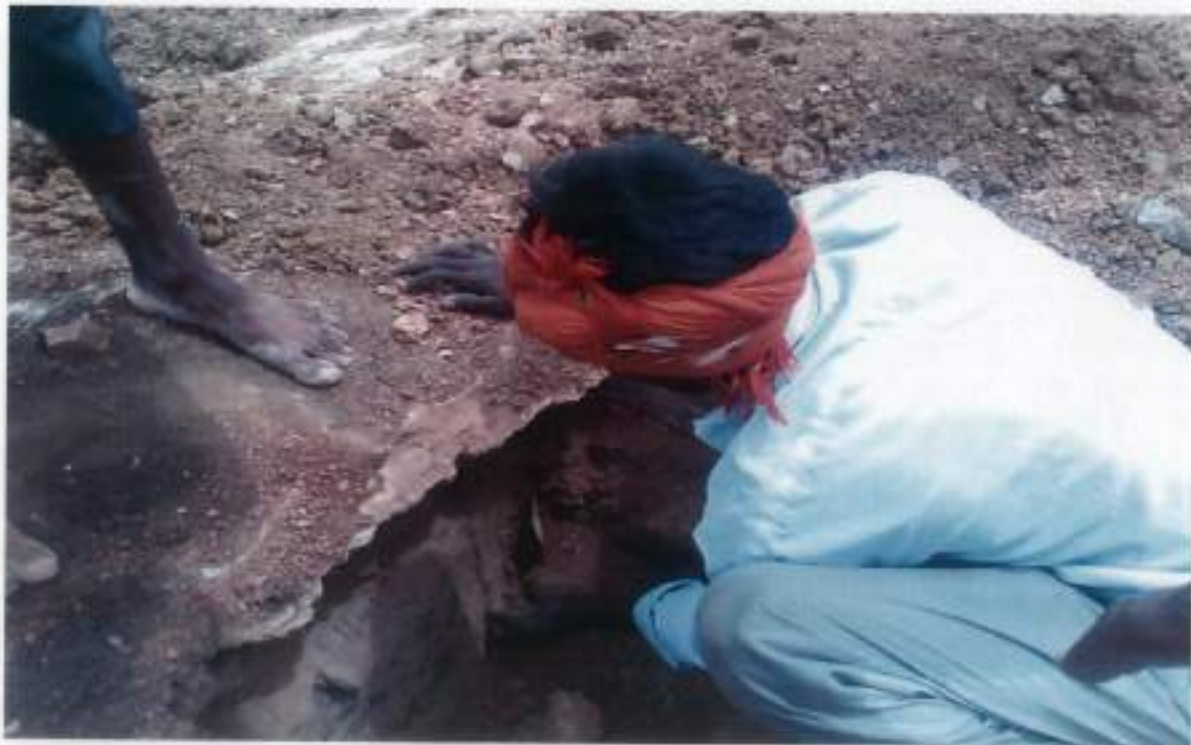
Tucked HDPE at the edge of the embankment
