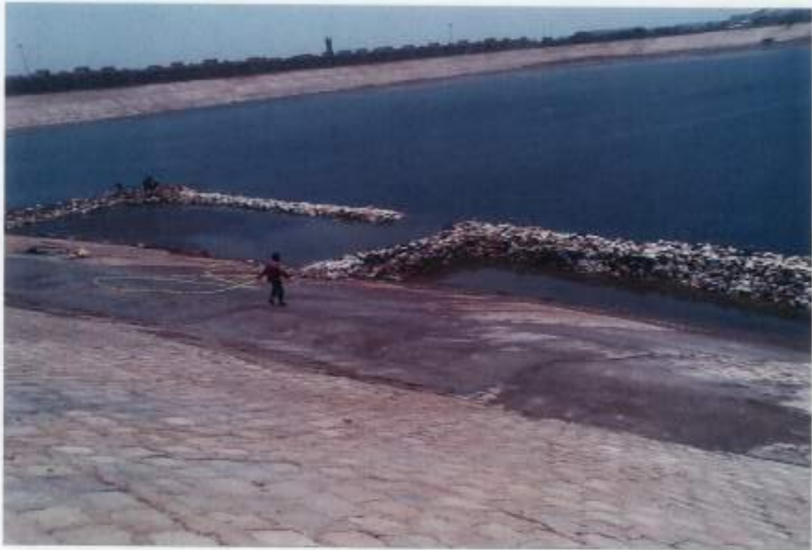
Rectification on upstream slope near intake structure Photo No-07
