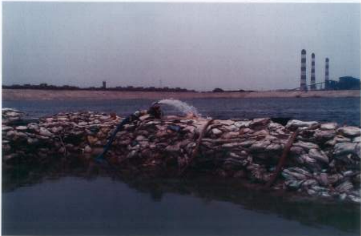
Dewatering at toe of the upstream side at intake structure
